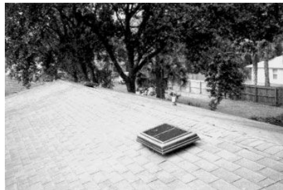
A case of misplaced effort. The solar panels built into the top of this attic exhaust fan mean energy-efficient cooling of a hot attic. But the fan can pull cool air from the house, cause back drafting, and introduce moisture problems.
